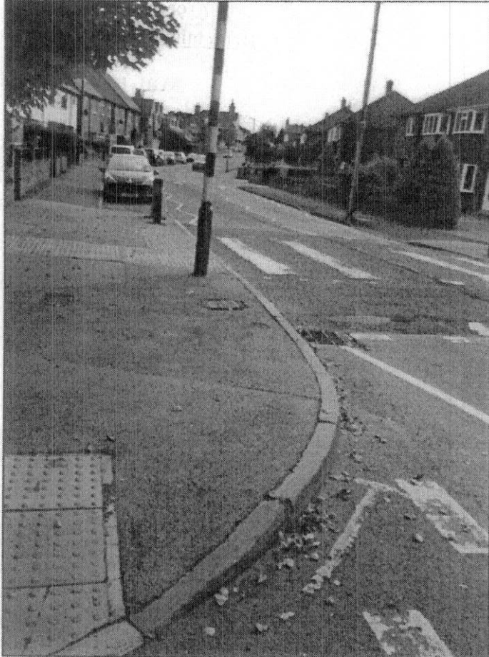
Kerb build-out outside Dringhouses Infant School
